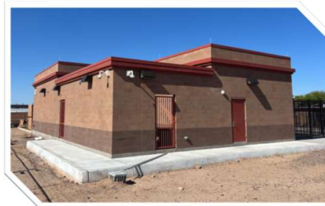
Traction Power Substation
