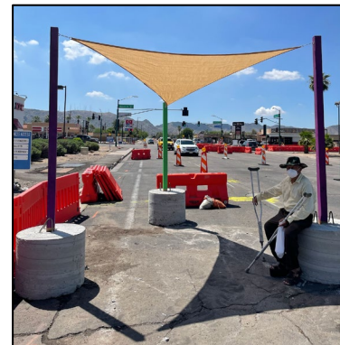
SCEDH Temporary Shade Structures
