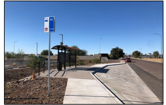
New Avondale Bus Shelter
