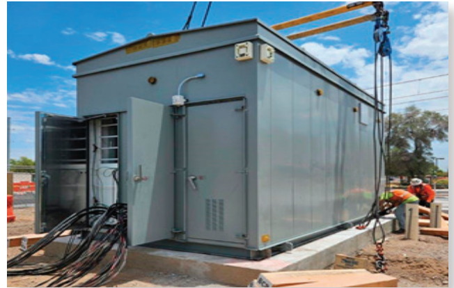
Installation of Mountain View Prefabricated Signals Building
