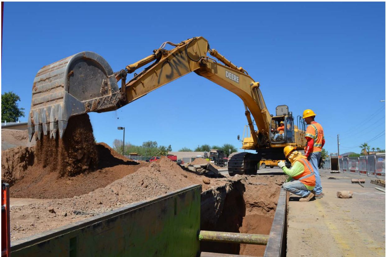
Northwest Extension – 19 th Avenue Utilities Relocation
