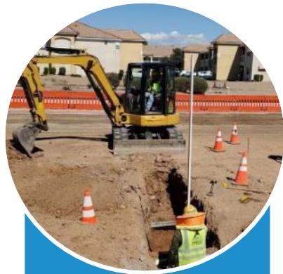
Underground Utility Relocation
